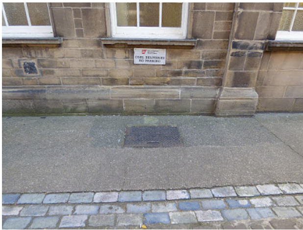
Coal hole at Wakefield Town Hall in Great Britain, 2018. (Stephen Craven CC BY-SA-2.0.)
